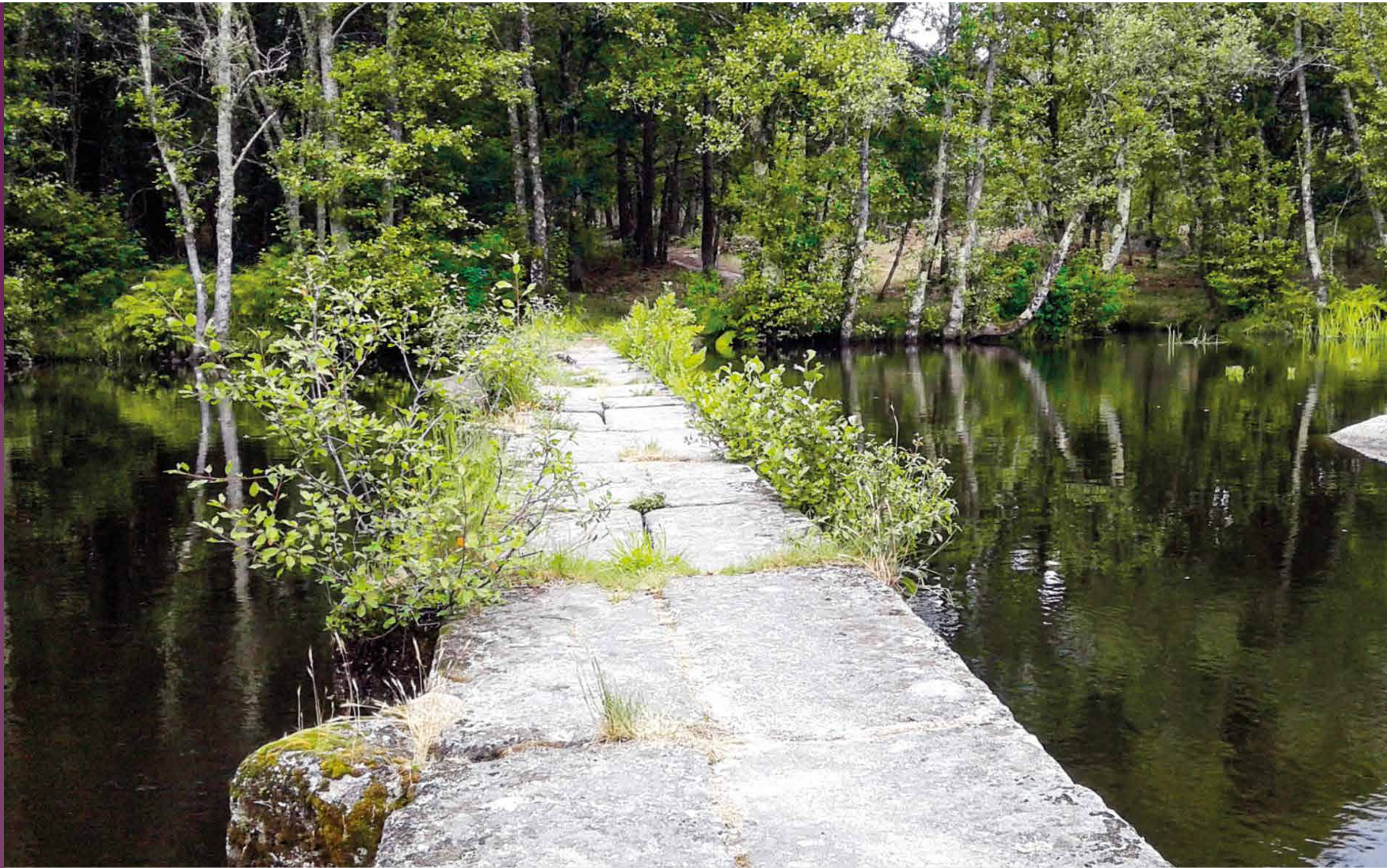
Ponte Pedonal - Torges / Pedestrian Bridge - Torges
